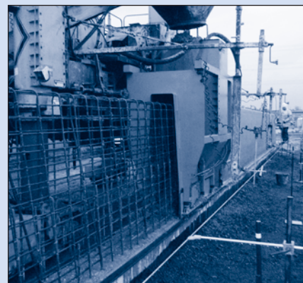
The cage reinforcement for the barrier wall was set in advance of the slipform paver and an open-fronted mould was used.
