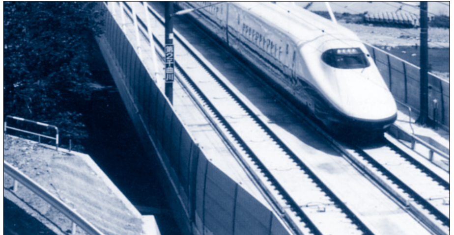
Concrete slabtrack in use for high speed trains in Japan
